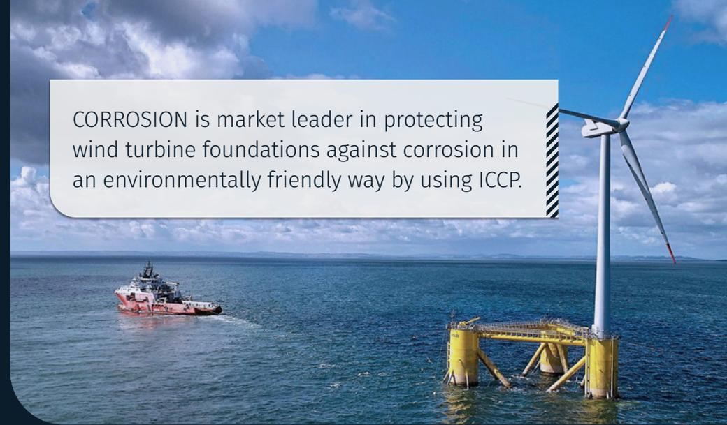
CP is a technique used to control the corrosion of a metal surface by making it the cathode of an electrochemical cell. This can be achieved in different ways. One way is to use a passive Galvanic Anode Cathodic Protection (GACP) installation system which uses aluminium anodes. However, this system is a major source of pollution due to the extreme amounts of anode material it deposits into the water as the anodes dissolve.
